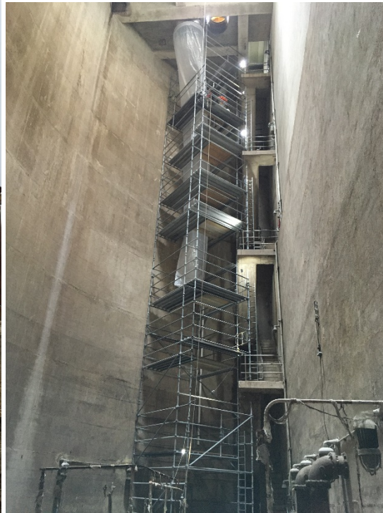
Wet well makeup air unit and exhaust fan; Installation of fabric duct on the east side of the wet well.
