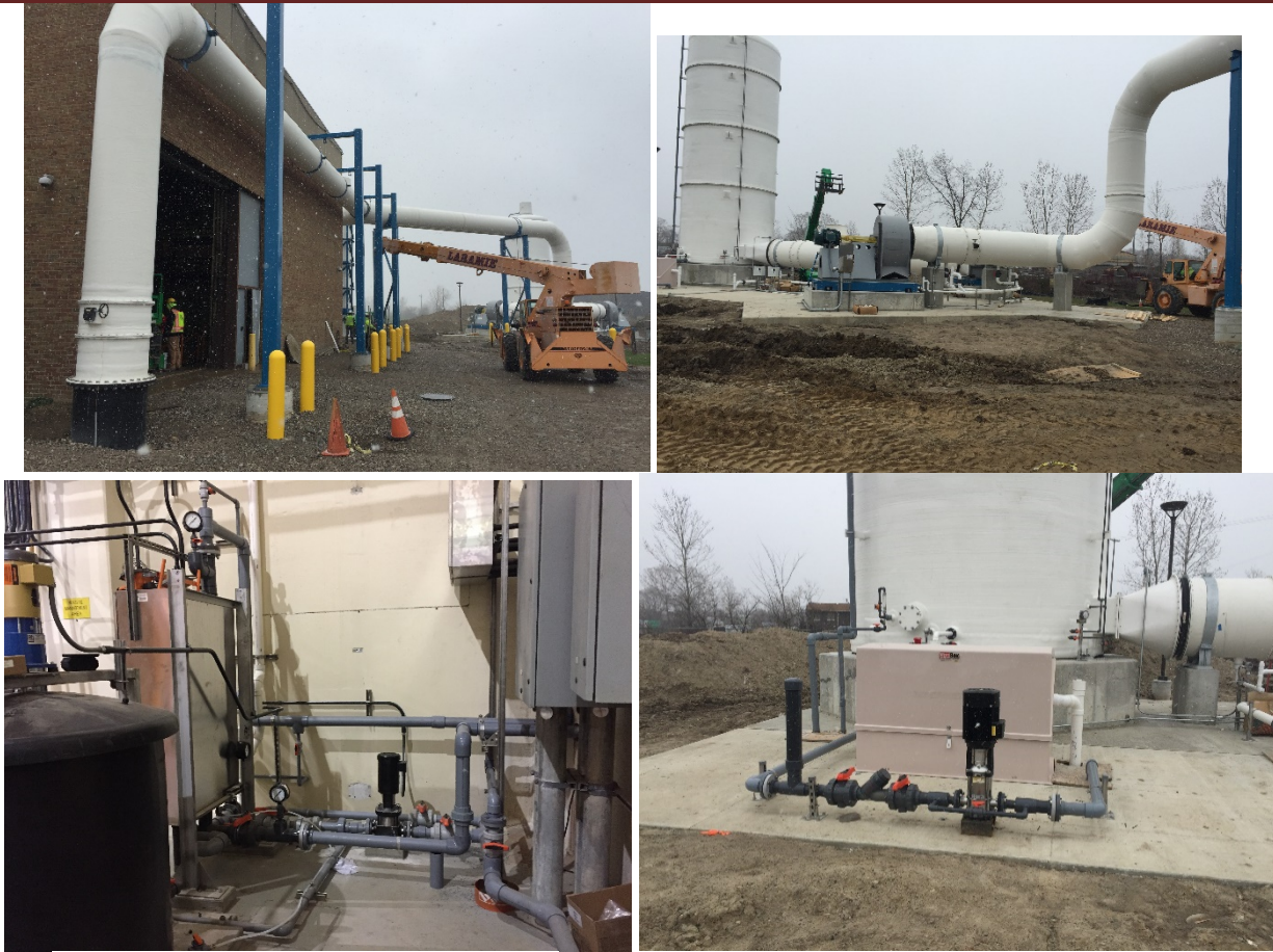
Installation of the FRP above ground duct sections leading to the BTF vessel; process water and drain piping including temporary startup system.
