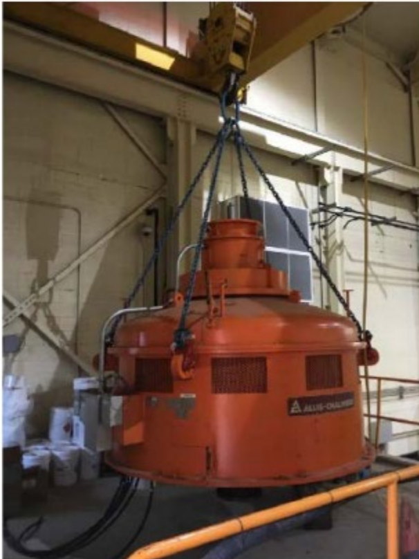
Removal of Pump No. 1 for repair.
