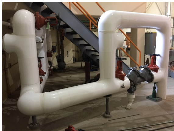
New 6-inch domestic water piping and insulation; DWSD supplied water meter.
