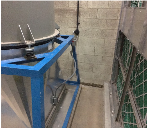
Power and controls conduit and wiring installation ongoing for HVAC system.
