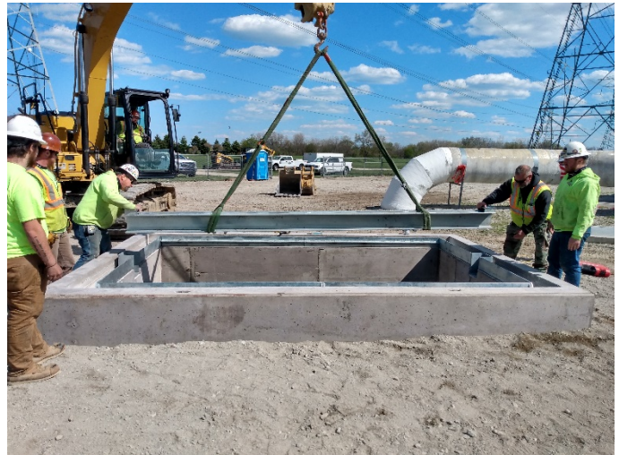
Removal of existing buried panels at CS-5 (upper left). Placement of midspan beam at CS-6 (above). Finishing grout work at CS-6 (bottom left).
