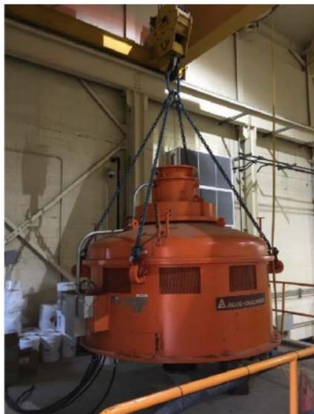
Removal of Pump No. 1 for repair.
