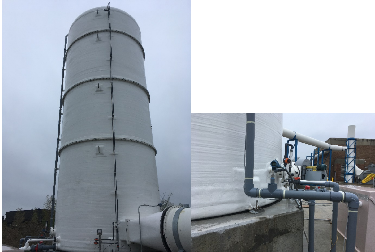
Installation of the process pipe labeling and heat tracing system for the biotrickling filter water and drain piping.
