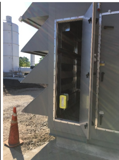
Wetwell make-up air unit dampers and actuator for HVAC system.
