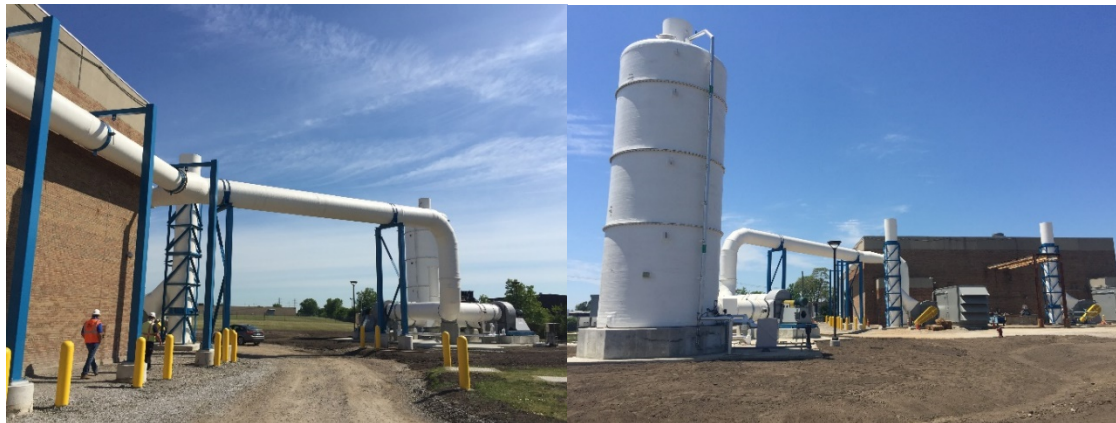
Biotrickling filter, FRP duct work, and wet well HVAC equipment along the north side of the Northeast Sewage Pumping Station.
