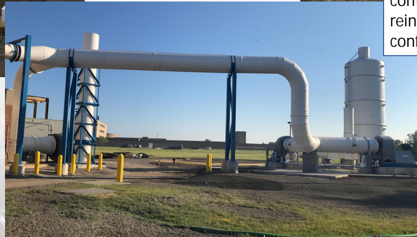
Fiberglass-reinforced plastic duct installation leading from the wet well and discharge chamber
