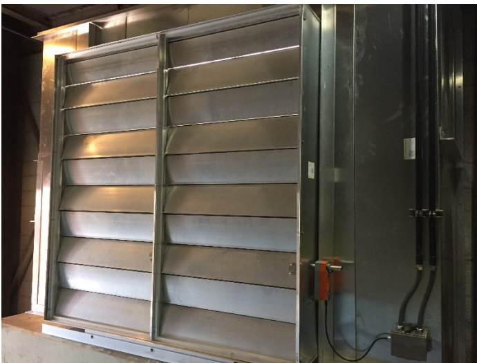
Drywell outside air modulating dampers and actuator for HVAC system.
