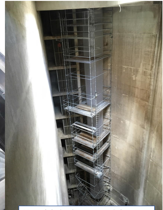
New fabric duct material conveys fresh air supply to the wet well on two sides
