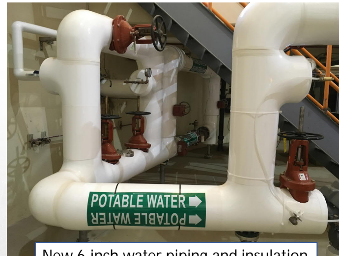
New 6-inch water piping and insulation
