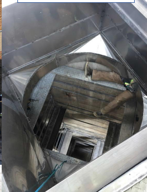
New stainless steel drop connection to fabric duct
