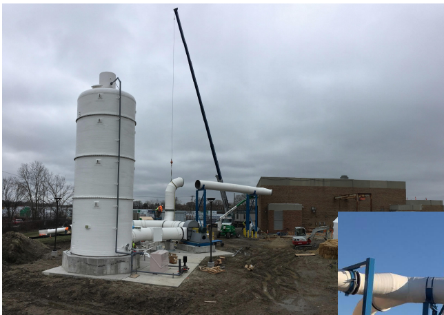
Fiberglass-reinforced plastic duct installation leading from the wet well and discharge chamber
