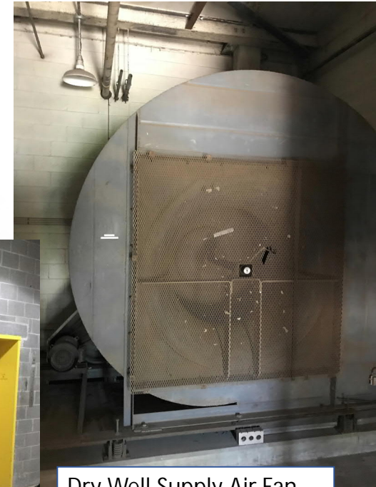
Dry Well Supply Air Fan
