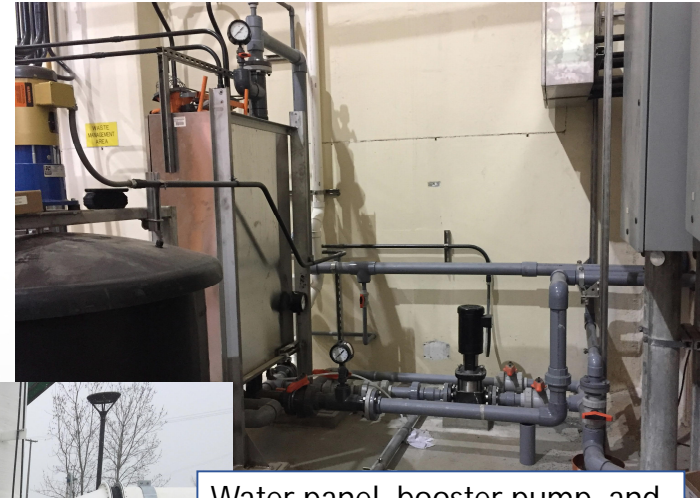
Water panel, booster pump, and process water and drain piping
