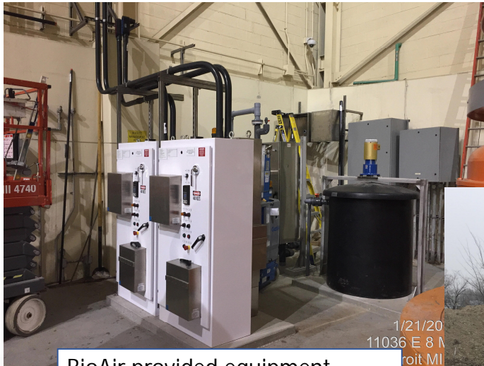
BioAir provided equipment including VFD panels, nutrient mixing tank, and water panel
