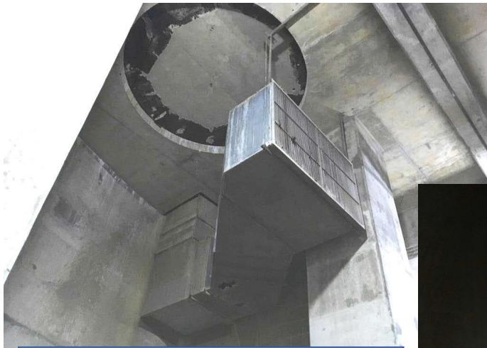
Dry Well Rectangular Supply Air Duct
