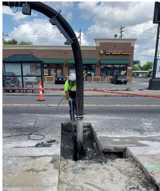
Potholing of Utilities at Proposed Shaft Location
