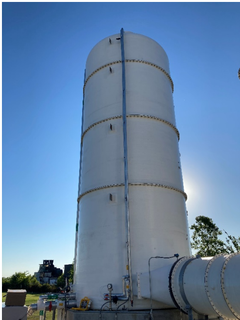
Biotrickling filter and associated sampling and testing equipment in place to monitor system performance.
