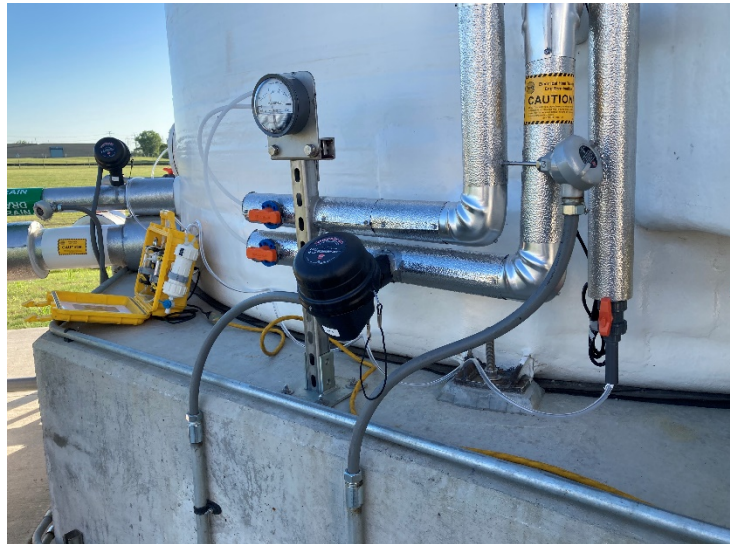
Biotrickling filter and associated sampling and testing equipment in place to monitor system performance.
