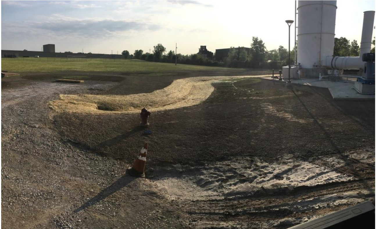
Turf restoration ongoing surrounding the new biotrickling filter.
