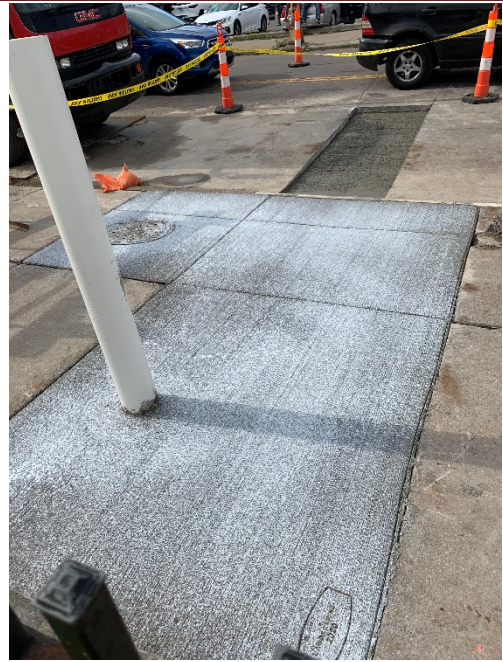
Restoration of site. PVC casing cast in place to guide future boring past utilities.
