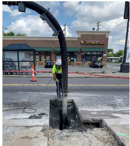
Potholing of Utilities at Proposed Shaft Location
