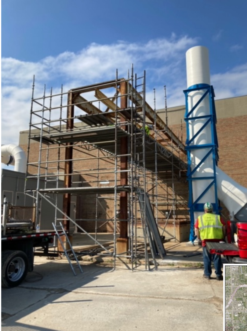
Scaffolding placement in preparation of 4-Ton crane replacement activities near the wet well.
