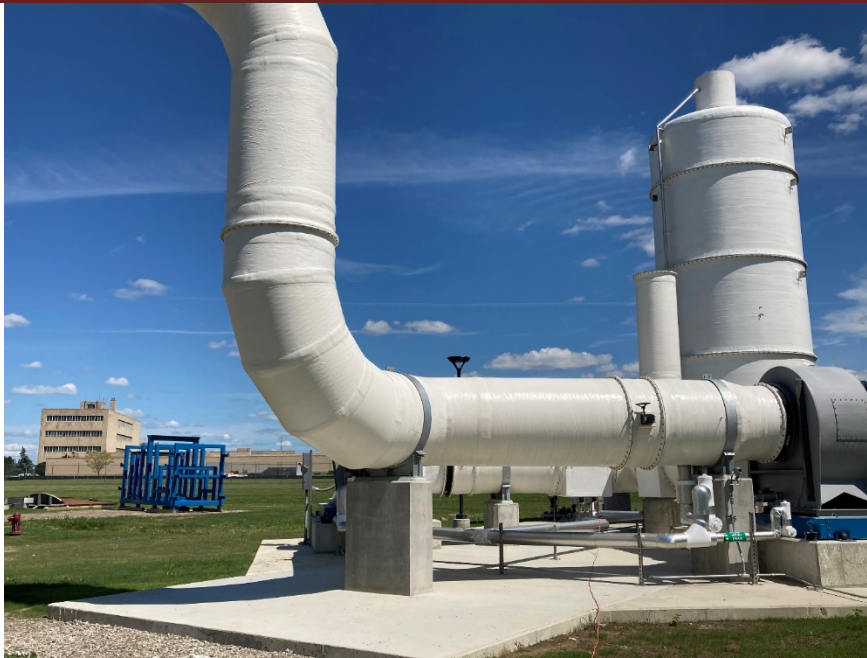
Biotrickling filter prepared and ready for performance testing activities.
