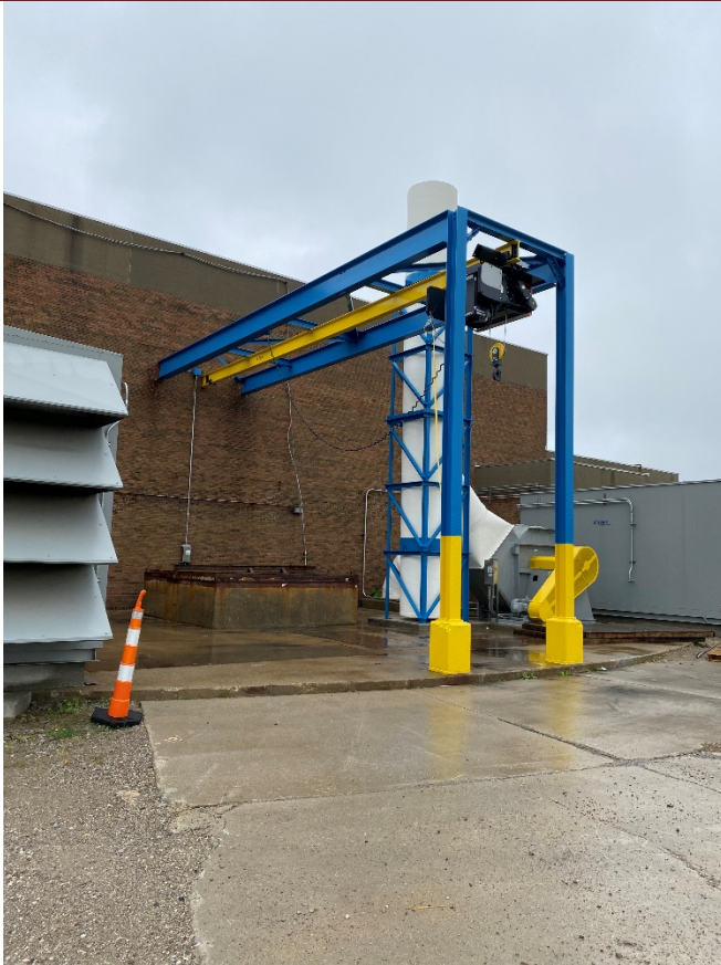
Finish coating and replacement of 4-Ton crane above the wet well.
