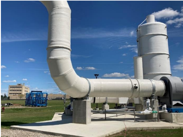
Biotrickling filter in full operational mode
