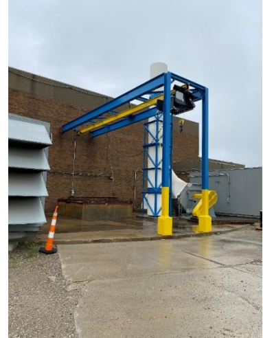
Finish coating and replacement of 4-Ton crane above the wet well.
