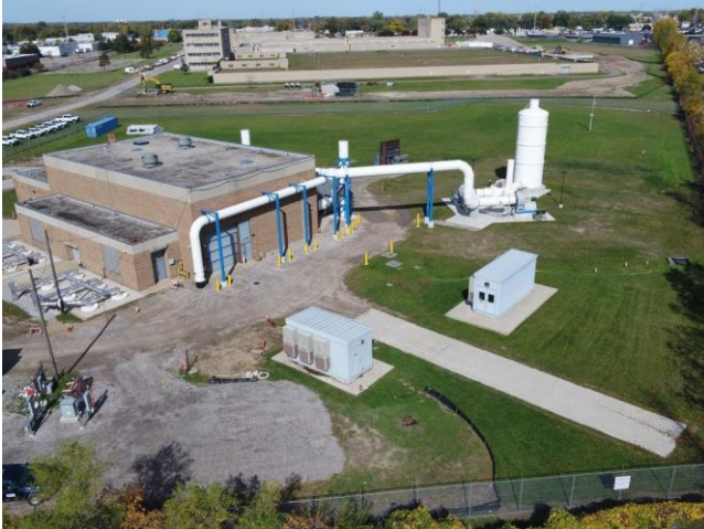
Biotrickling filter in full operational mode
