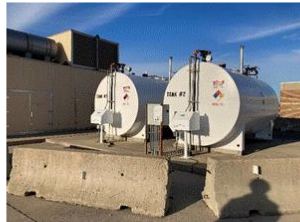
NESPS Fuel Tank Rehab (paint, fittings, fuel lines, etc.)
