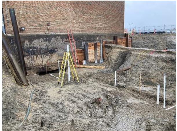
Temporary Earth Retention System near existing transformer bay
