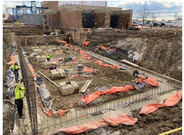
NESPS Refurbishment spread footing construction
