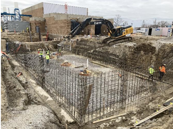
NESPS Electrical Building Slab and Wall Installation
