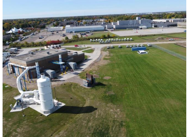
Biotrickling filter in full operational mode
